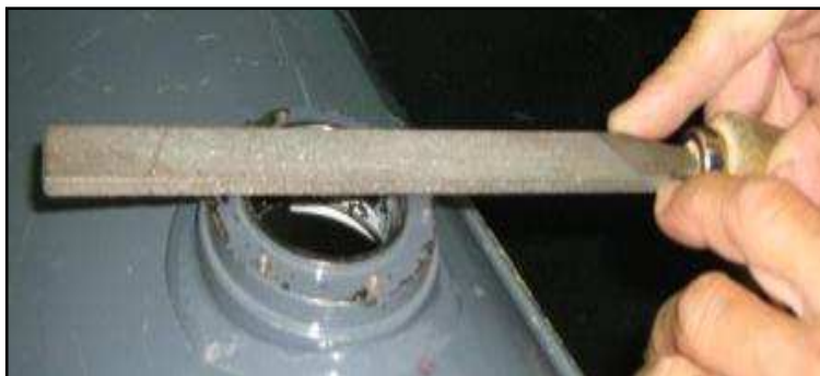
Figure 4: Removing of the paint from the seat ring of the tank
